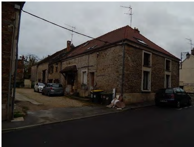
Cour commune, Grande rue
